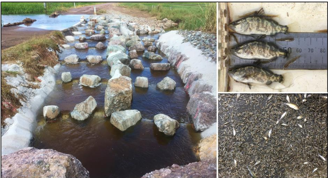
Figure 15. A rock ramp fishway constructed to remediate a road causeway (water surface drop) on Tedlands wetlands in Koumala, central QLD (left). Young of the year Barramundi recruits captured successfully ascending the fishway during post-construction monitoring (top right). This is the typical size of juvenile Barramundi undertaking life-cycle-dependent migrations from saltwater to freshwater. Thousands of juvenile Empire Gudgeon (and a few Barramundi) were recorded in a single trap set successfully ascending the fishway (bottom right). These Empire Gudgeon and Barramundi were migrating from saltwater to freshwater.
