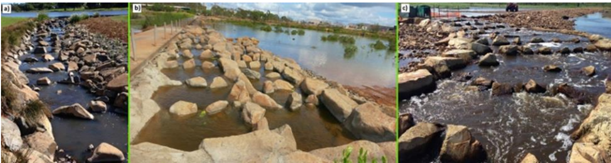
Figure 16. Nature like rock-ramp fishways: a) Full width (Gooseponds Ck, Mackay), b) Dog-leg (Lake Callemondah, Gladstone) c) Partial width (Tedlands Ck, Koumala)
