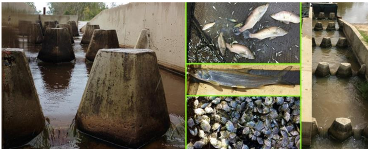
Figure 17. Concrete cone fishway on Boundary Creek, Koumala; showing fish successful at ascending, top to bottom; juvenile Barramundi and Empire Gudgeon, Giant Herring & over one thousand juvenile Banded Scats & Threadfin Silver Biddy.
