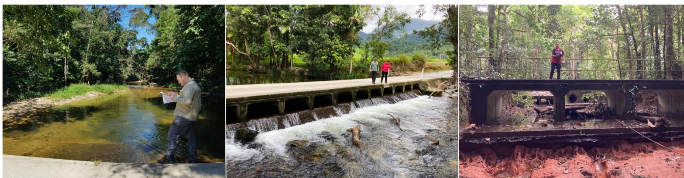
Figure 9. Examples of typical fish barriers validated during ground-truthing by Terrain NRM (Lana Hepburn & Tom Crow), Wet Tropics Waterways (Richard Hunt and James Donaldson), and Catchment Solutions (Matt Moore) staff. From left to right; Causeways on Whyanbeel Creek (BarID:1278, Rank:21), Saltwater Creek (BarID:1218, Rank:14), and a tributary of Hutchinson Creek (Daintree Basin) (BarID:1801, Rank:56).
